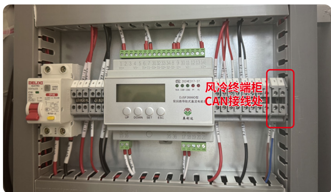
(风冷终端通信CAN图)
